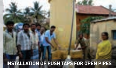
INSTALLATION OF PUSH TAPS FOR OPEN PIPES
