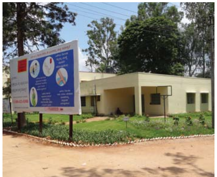
Primary Health care premises at Bidadi after restoration
