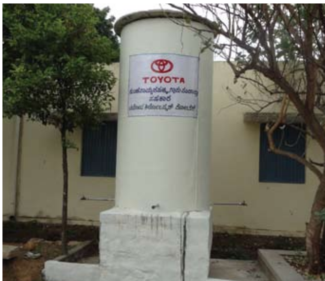
Water storage tanks built at villages
