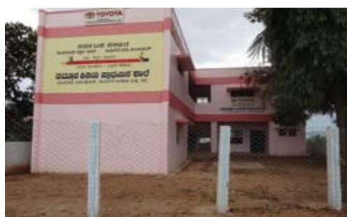
Medanahalli Government School constructed by TKM
