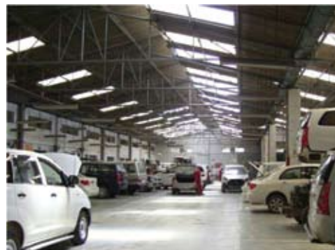
Daylight Harvest using transparent Fibre Glass sheet at Toyota, Gurgaon
