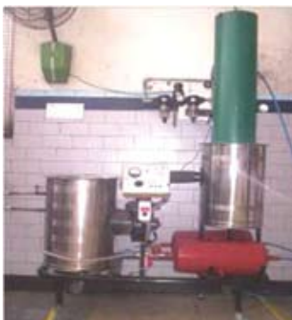
Installation of Automatic Air Filters at Radiant Toyota, Ludhiana
