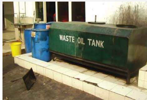
Safe collection & Recycling of Waste Oil Plant
