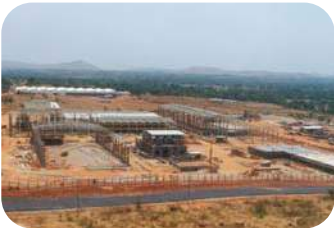
1997 Construction of TKM
