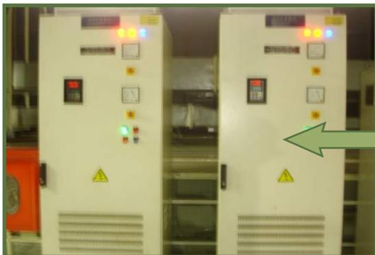
Fig 5.5: VFD installed at Paint Shop to optimize the electricity consumption ultimately yielding 12% reduction
