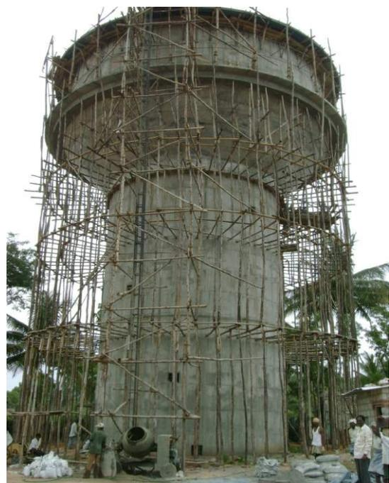
Fig 10.1: Construction of Water Tank
