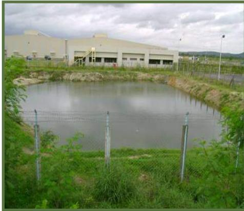
Fig 6.6: Rain Water Harvesting Pond
