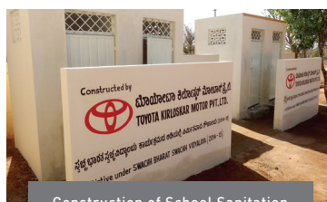
Construction of School Sanitation Units in Government Schools
