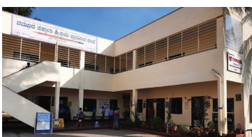
Modernisation of the Government Schools Infrastructure & Learning Improvements
